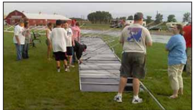
Storm brought the wall down at Salute to Troops. Volunteers helped put it back up.
